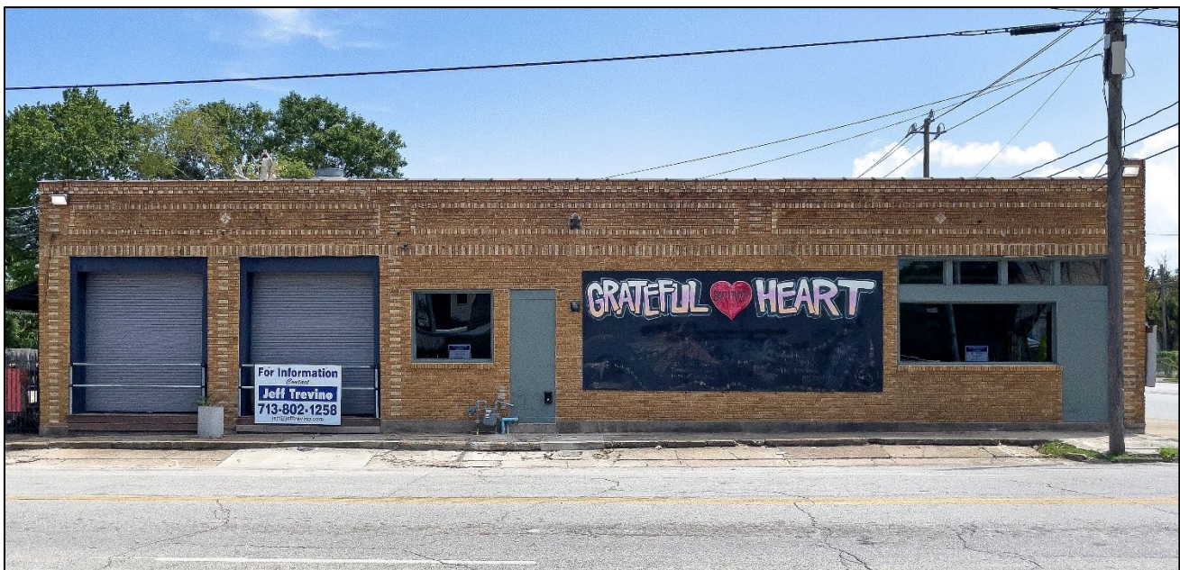
SIDE FAÇADE FACING CROCKETT STREET PHOTOS BY JIM PARSONS, PRESERVATION HOUSTON
