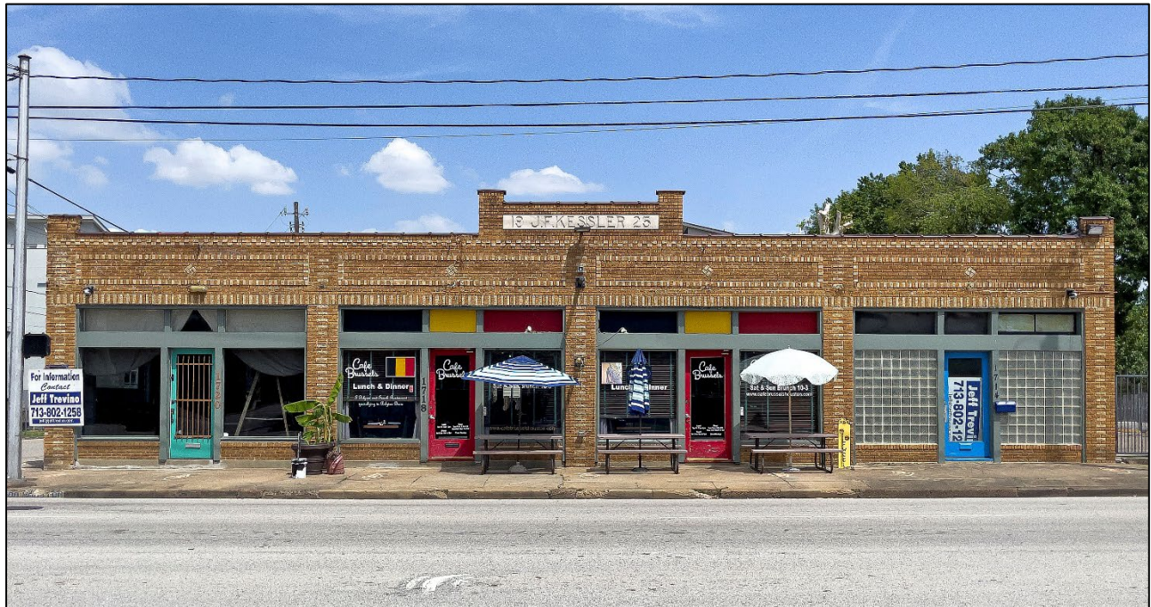
FRONT FAÇADE FACING HOUSTON AVENUE
