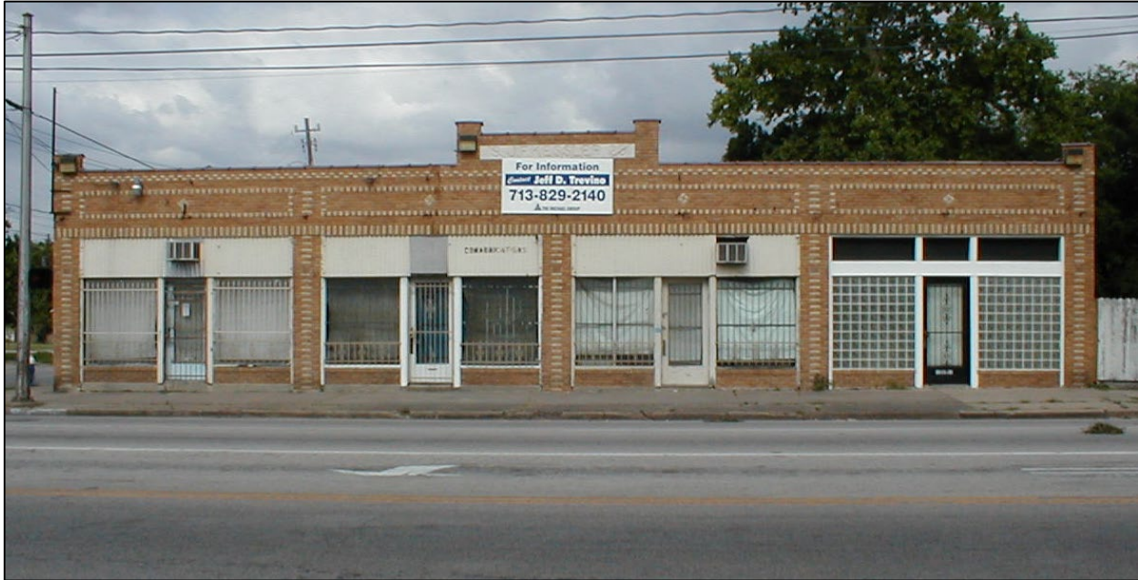
FRONT FAÇADE FACING HOUSTON AVENUE
